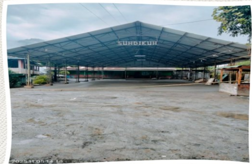
Sihdi Kuh Floor Casting
